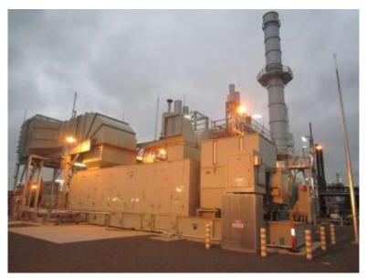
This baseload cogeneration plant provides steam and electricity to the Qenos' manufacturing plant. In addition to baseload supply it also has the capability to disconnect from the distribution network at times of fault and operate in 'Island Mode' to sustain site operation.
